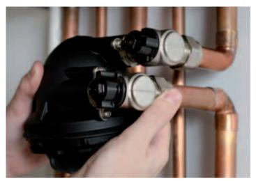
**3.** Slide the system filter onto the pipework and hand tighten, following the flow direction indicated on the isolation valves.
