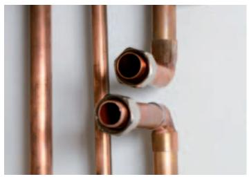
2. Measure, mark and cut out a 70mm section of pipe. The two copper elbows are different, the shorter elbow is fitted on the pipe that returns to the boiler. Prepare the elbows supplied and solder onto the ends of the pipes.
