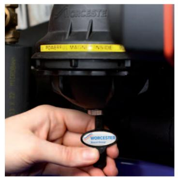
**2.** Open the bottom of the filter with a radiator bleed key to relieve any pressure from the body.
