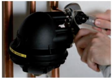
**4.** Tighten the compression fittings firmly, but do not overtighten. Then, using a suitable spanner, open the isolation valves. This will then allow you to refill the heating system and run the central heating system and check for leaks.
