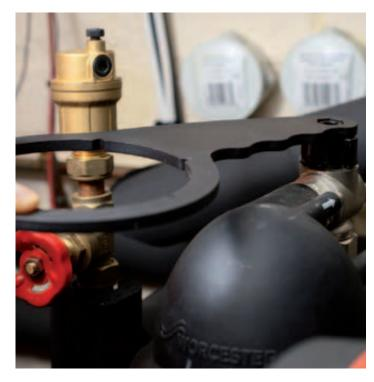
1. Simply isolate the filter before servicing.
