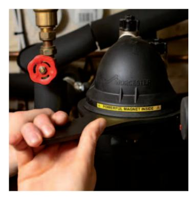
**3.** The specially supplied spanners are used to open the filter.
